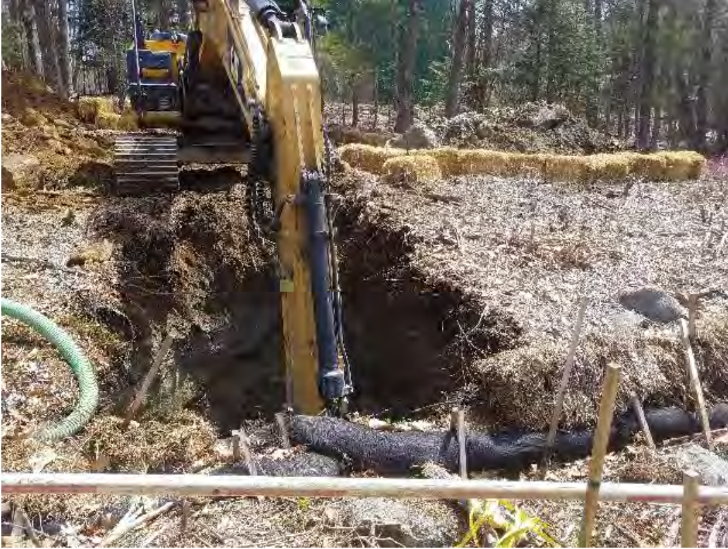
Fig 19: Excavating foundation for Str. 34. Viewing east. (04-29-20).
