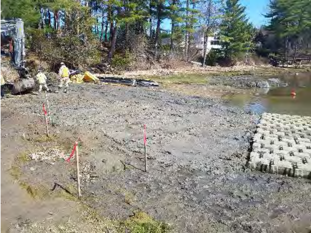
Fig 25: Concrete blocks installed in tidal flat and backfilled with native material at Gundalow landing/east side of the Bay. Viewing southeast. (04-21-20)
