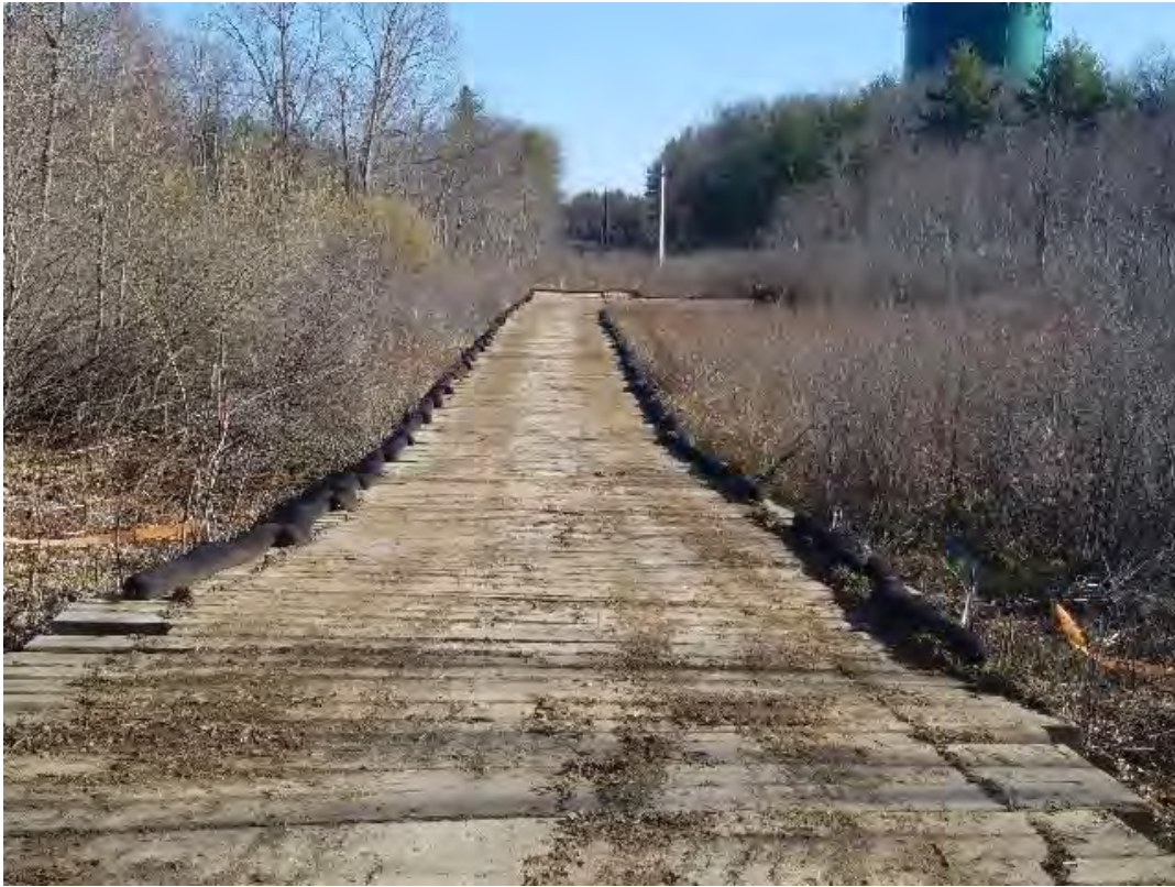
Fig 1: Access road to Str. 35, through wetland DW41. Viewing north. (04-23-20).
