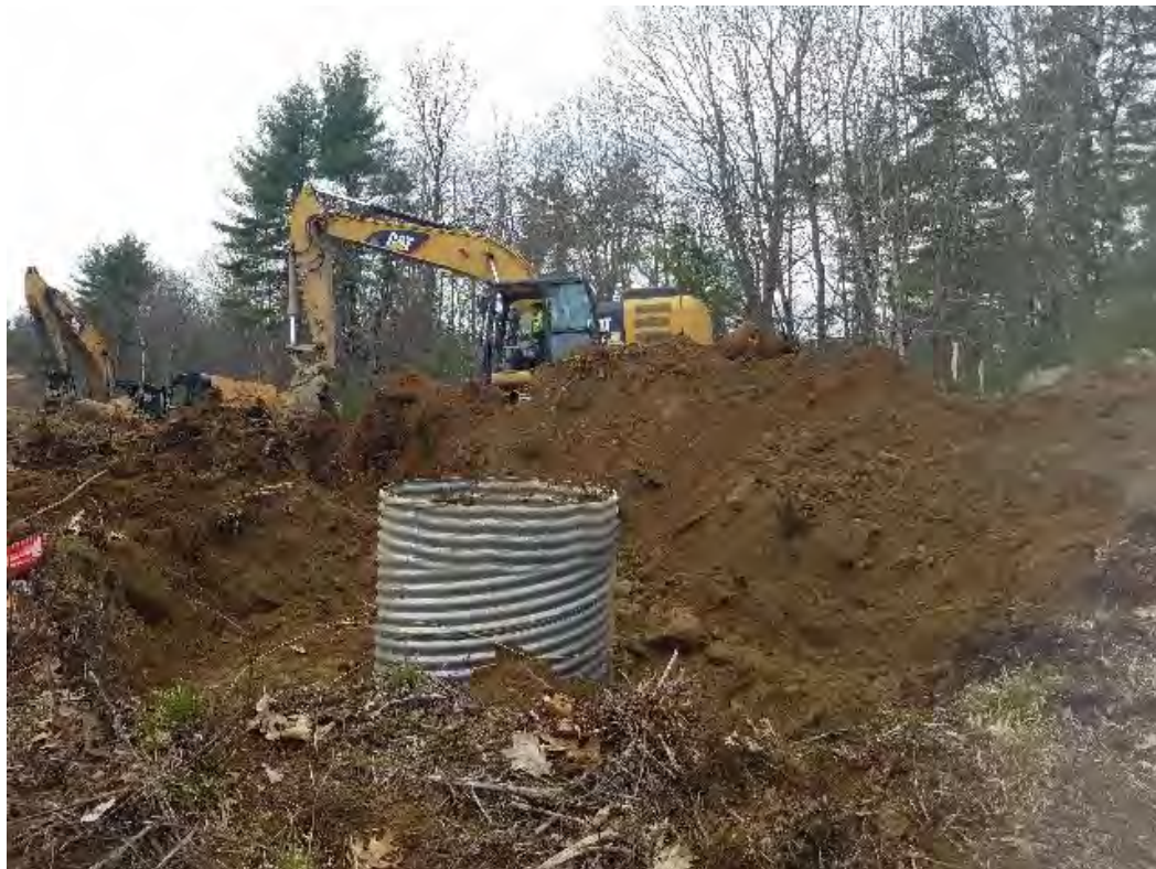
Fig 18: Setting foundation can for Str. 41. Viewing south. (04-28-20).
