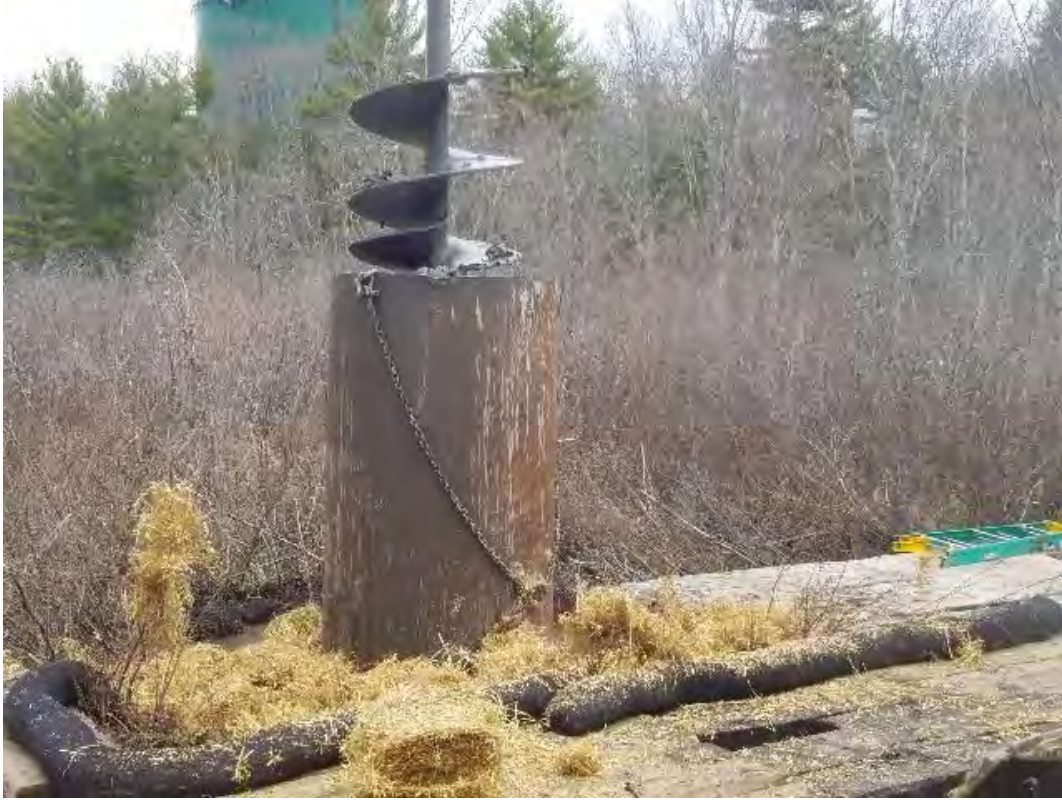
Fig 11: Excavating Str. 35 using hard can and auger. Viewing north. (04-25-20).
