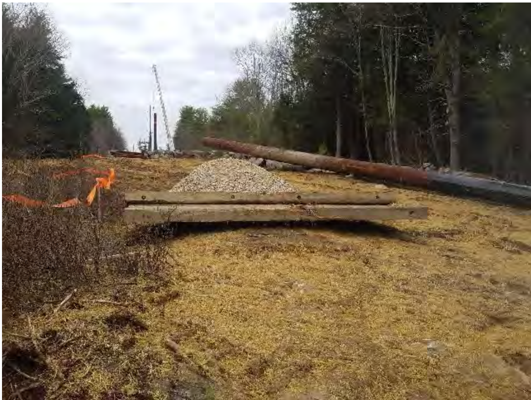
Fig 8: Str. 83 foundation can set and work area. Viewing west. (04-25-20).
