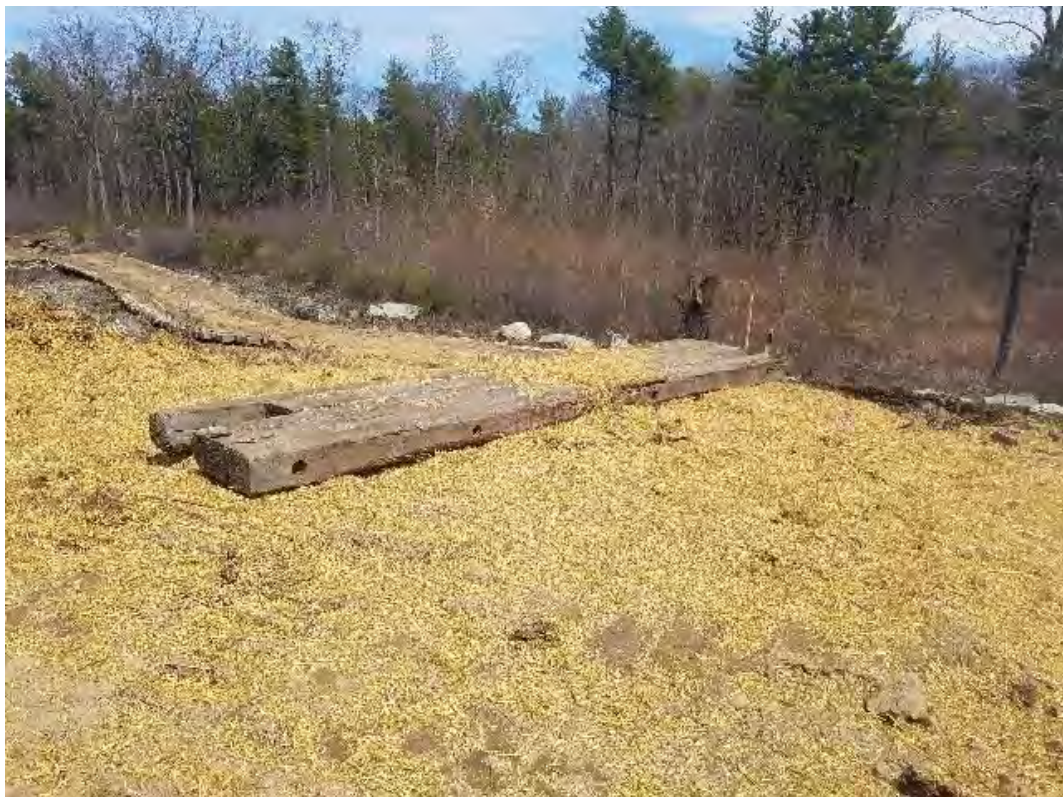
Fig 20: Str. 41 foundation can set. Viewing north. (04-29-20).
