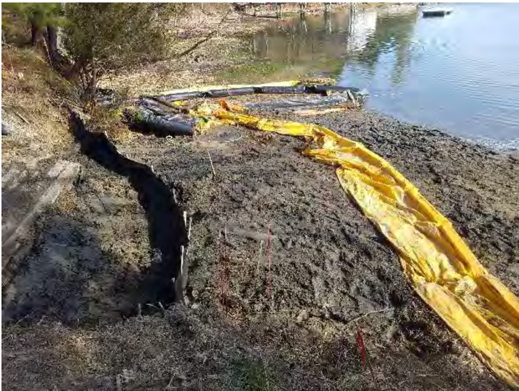
Fig 26: BMPs installed in intertidal zone at end of day at Gundalow landing/east side of the Bay. Viewing southeast. (04-29-20).
