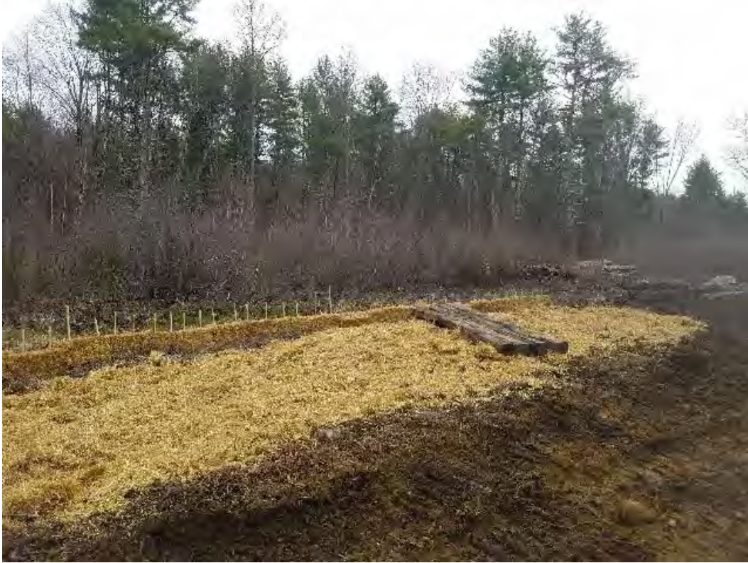
Fig 17: Str. 39 foundation can set. Viewing east. (04-28-20).
