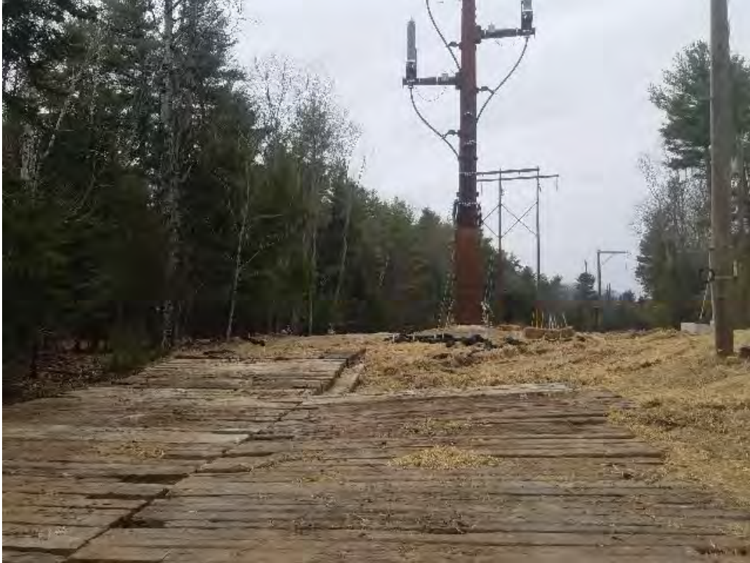
Fig 7: Crew installed timber mats for wire pull pad at Getchell property/west side of the Bay. Viewing west. (04-24-20).
