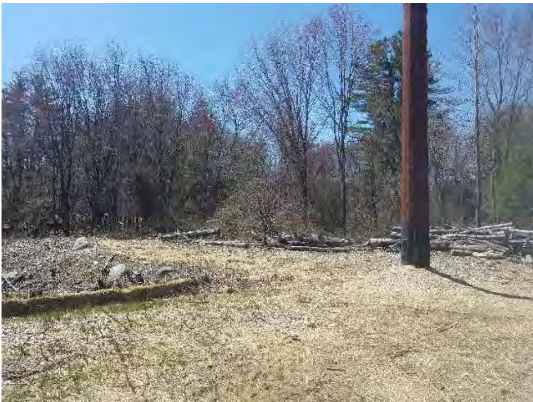
Fig 2: Str. 127 pole set and work area. Viewing south. (04-23-20).
