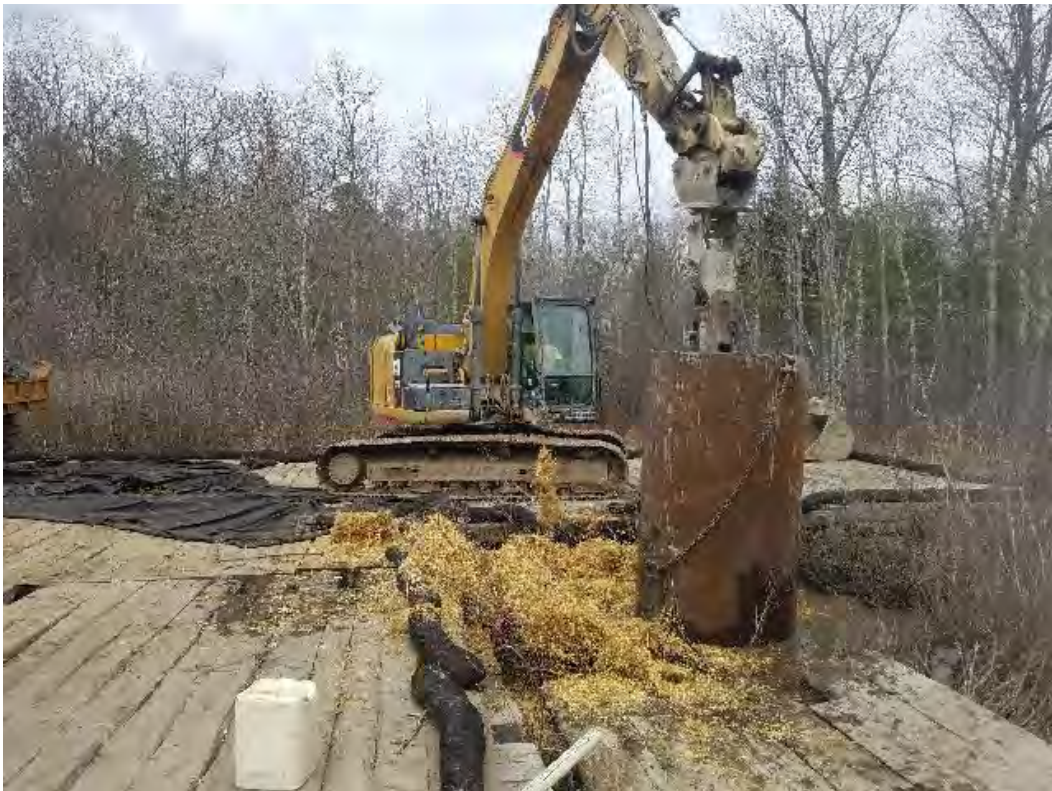
Fig 12: Excavating Str. 35 using hard can and auger. Viewing west. (04-25-20).
