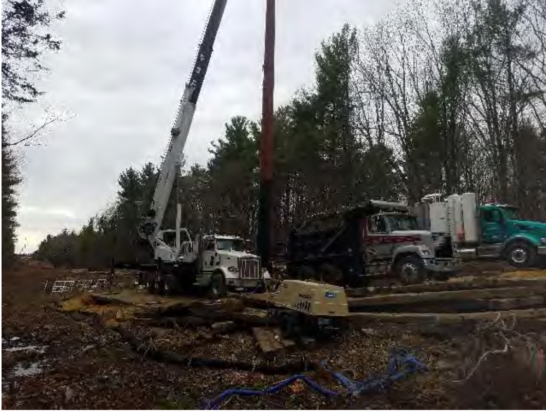
Fig 9: Crew raising Str. 89 pole. Viewing southeast. (04-25-20).
