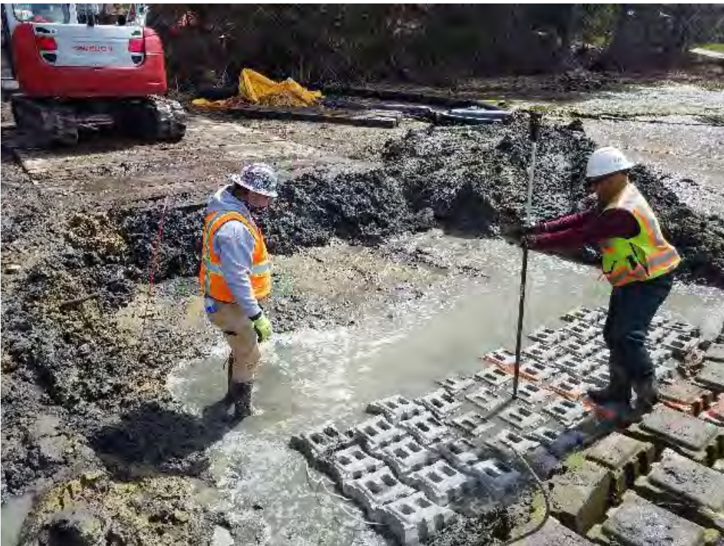
Fig 24: Blu Roc burying concrete blocks in tidal flat for cable protection at Gundalow landing/east side of the Bay. Viewing southeast. (04-29-20).
