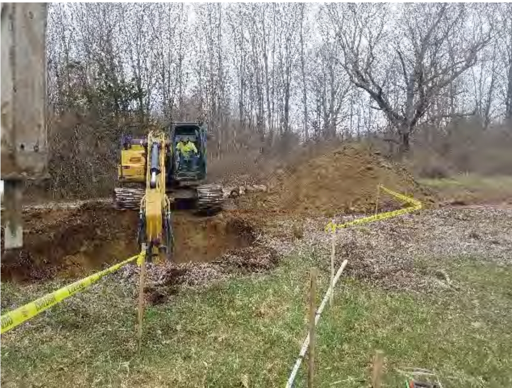
Fig 4: Excavating foundation for Str. 38. Viewing east. (04-24-20).
