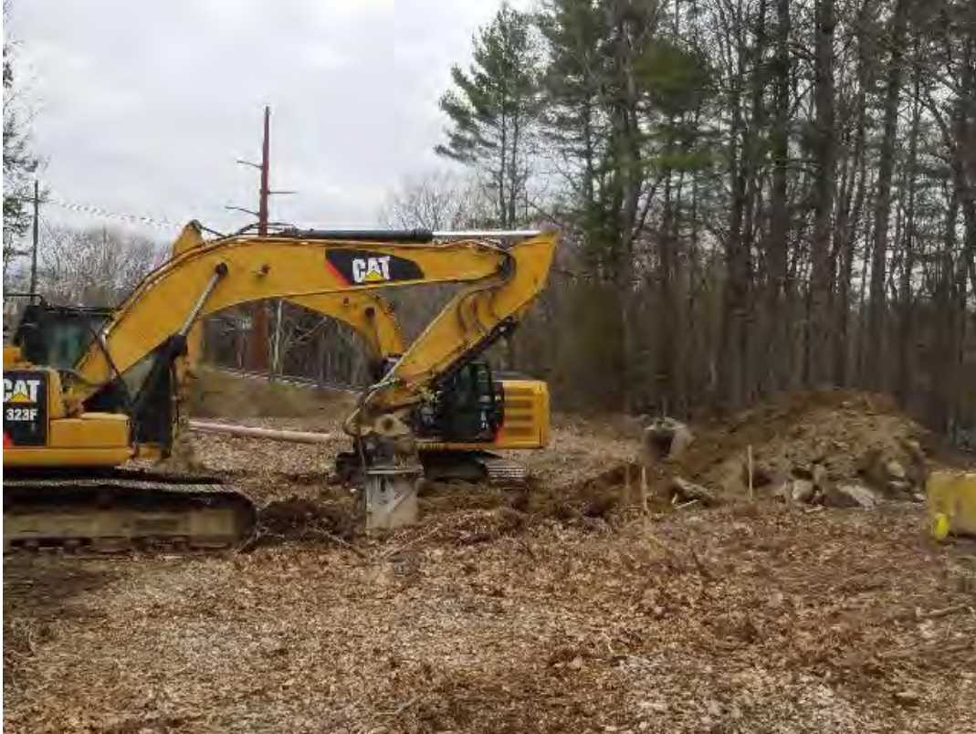
Fig 13: Hammering ledge for foundation at Str. 33. Viewing north. (04-25-20).
