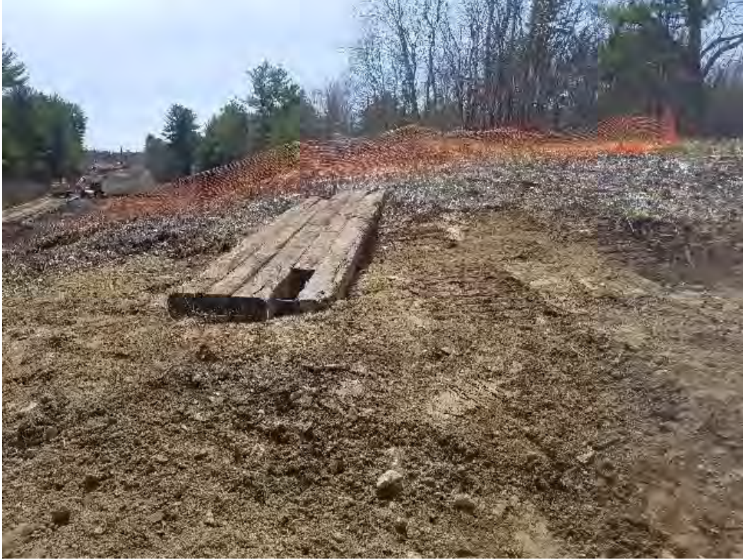
Fig 21: Str. 43 foundation can set. Viewing south. (04-29-20).
