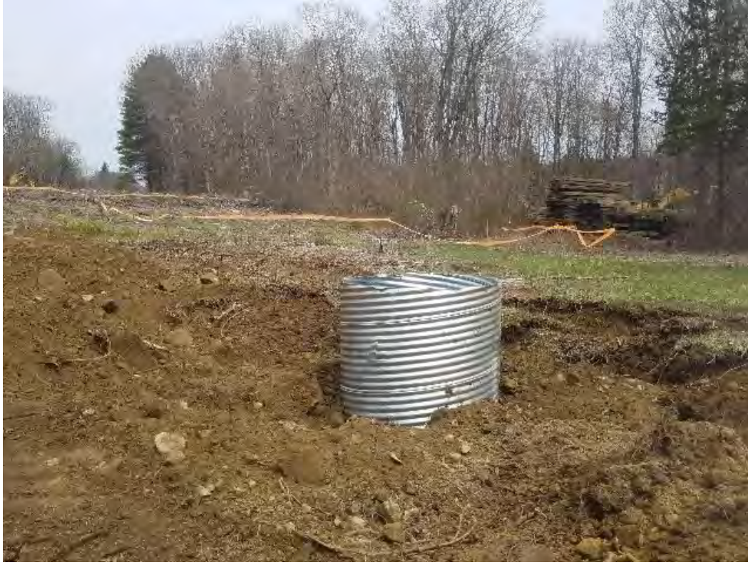
Fig 5: Foundation can set for Str. 38. Viewing northeast. (04-24-20).
