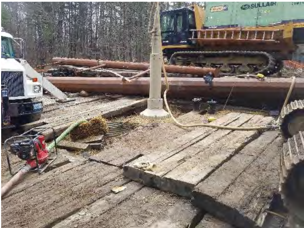
Fig 16: Pumping groundwater out of Str.89 foundation hole. Viewing south. (04-28-20).
