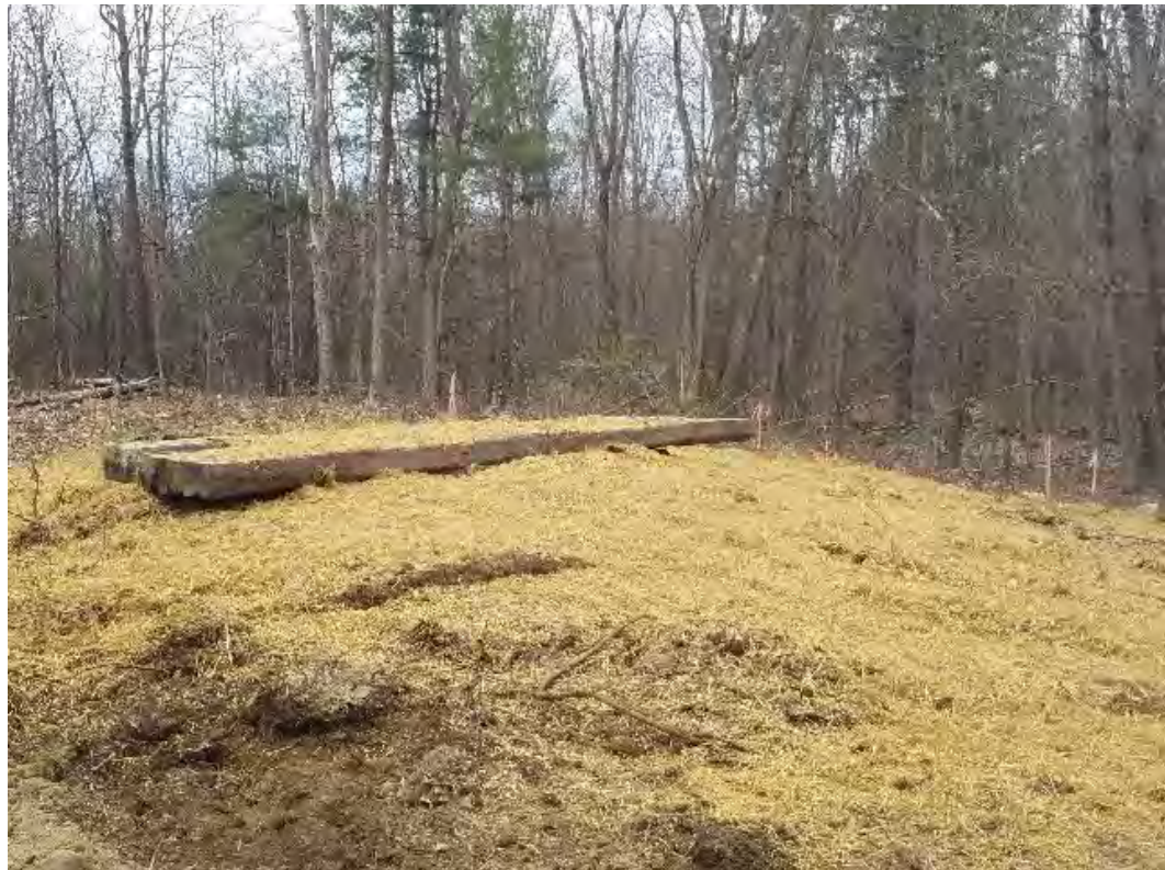
Fig 10: Foundation can set for Str. 41 and work area. Viewing west. (04-24-20).
